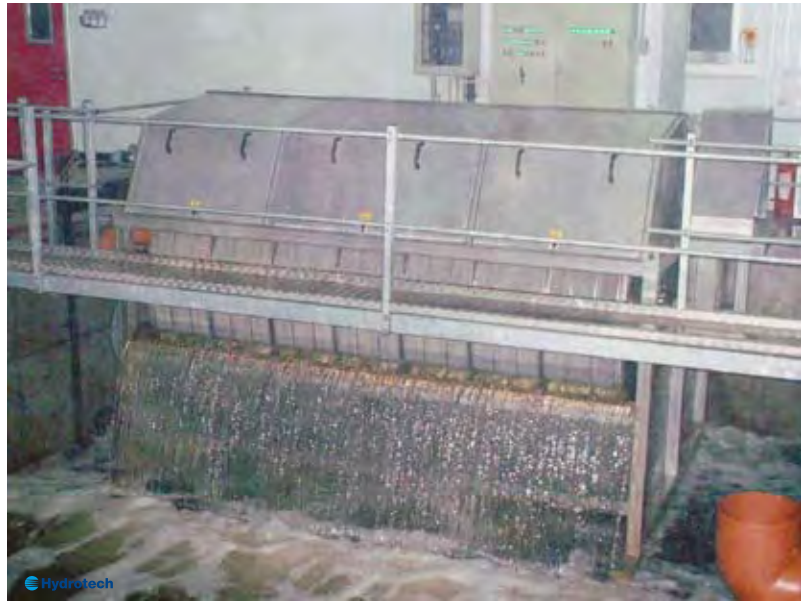
Hydrotech Drumfilter installed at a recirculating salmon farm.
